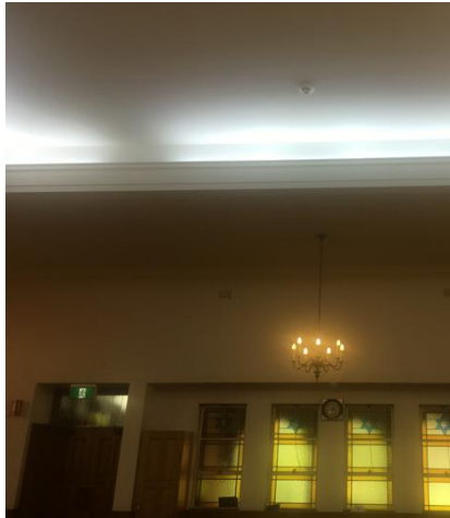
Internal ceiling detail.
